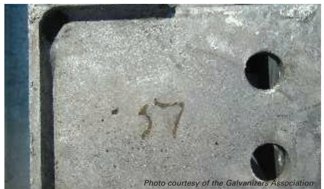
Photo courtesy of the Galvanizers Association
