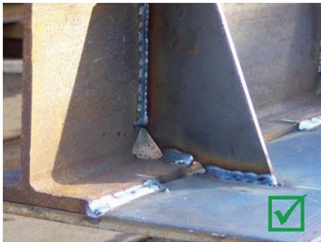
The flanges on this beam have been cropped before welding into place. Cost effective and excellent venting. Well done!
